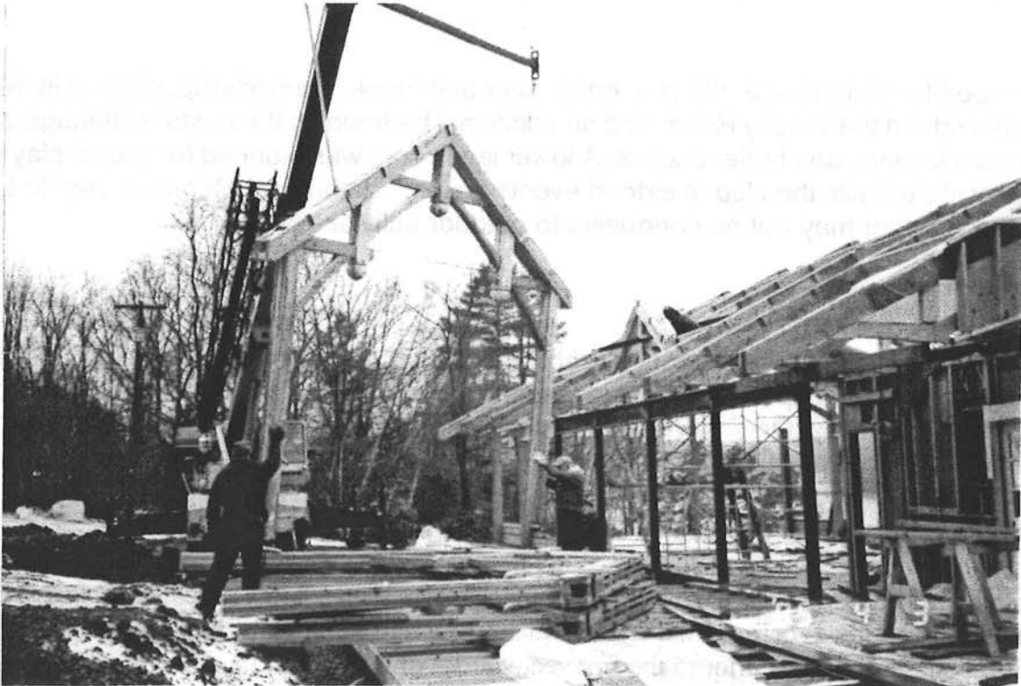
Adding the new entrance
